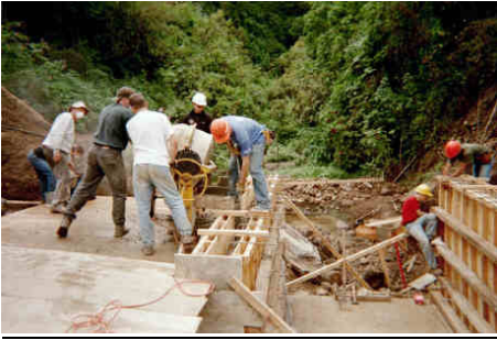
2004 Guatemala Bridge Project
